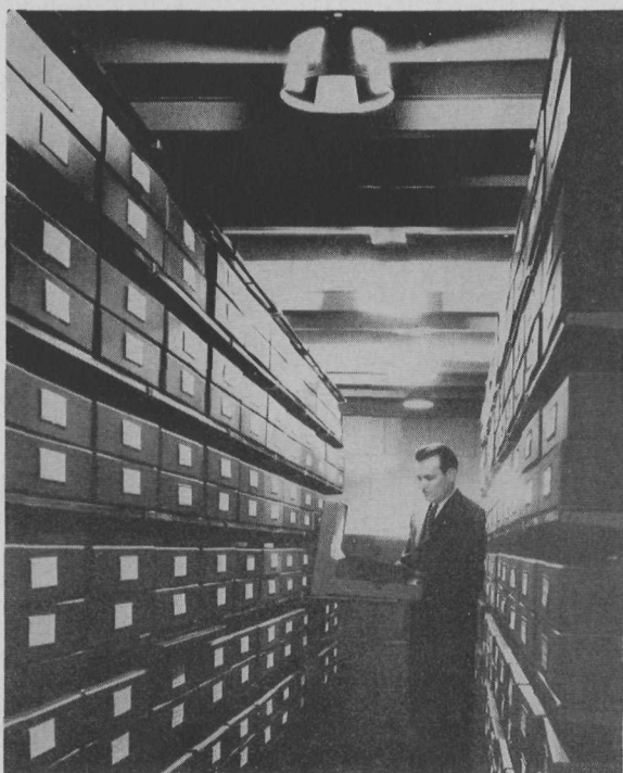
FIGURE II VIRGINIA STATE LIBRARY Shows a portion of a range of 12 inch shelves in use. The sliding reference shelf is also illustrated
