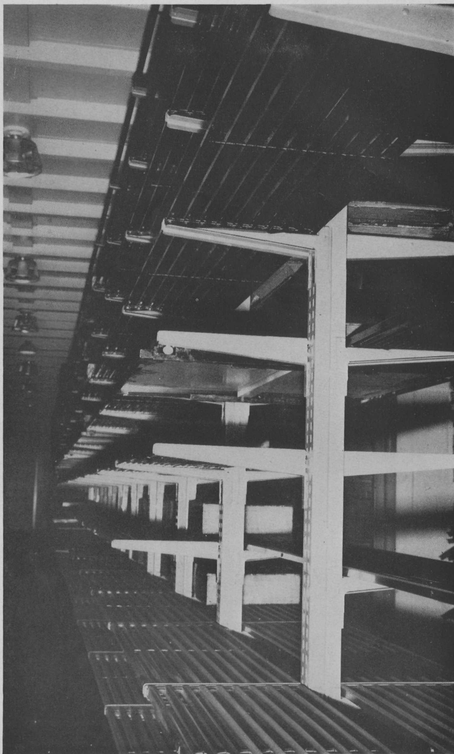
FIGURE I VIRGINIA STATE LIBRARY Shows the cantilever arrangement whereby the shelves are engaged to the columns.
