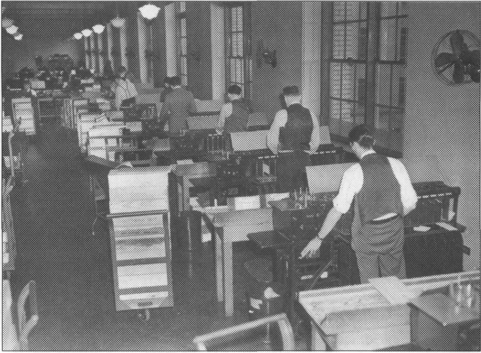
The machines in this undated photograph from the Bureau of the Census appear to be examples of one type of electrical sorting box , referenced in text note 3. The caption that accompanied the photograph says that the “machine is a mechanical sorter which is used by the United States Census Bureau in its tabulation system. The machine sorts cards automatically into different classifications as may be required.” Photograph 29-CM-E-16. Records of the Bureau of the Census, Record Group 29; The National Archives at College Park, Maryland.
